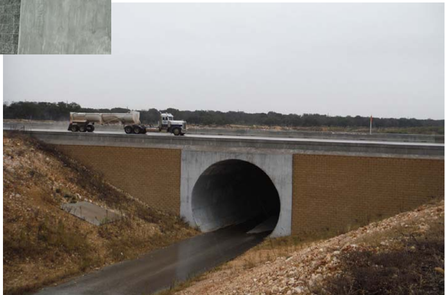
Seattle WA: 3,000m 2 of modular block retaining wall as part of new road interchange. Maximum wall height 8m.
