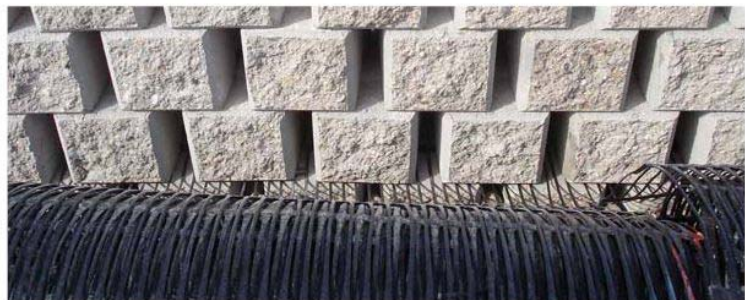
View of the wall the side of backfill
