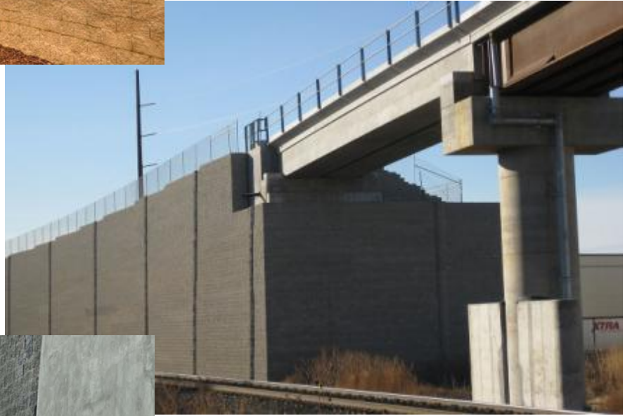
Seattle WA: 3,000m 2 of modular block retaining wall as part of new road interchange. Maximum wall height 8m.
