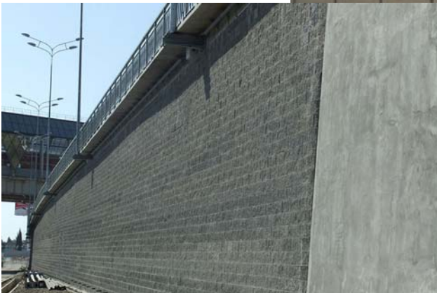
Seattle WA: 3,000m 2 of modular block retaining wall as part of new road interchange. Maximum wall height 8m.
