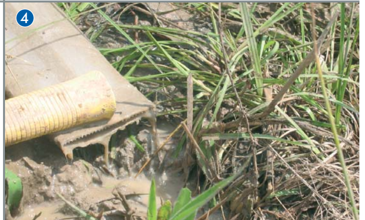
Drive Plati-Drain® into optimum position
